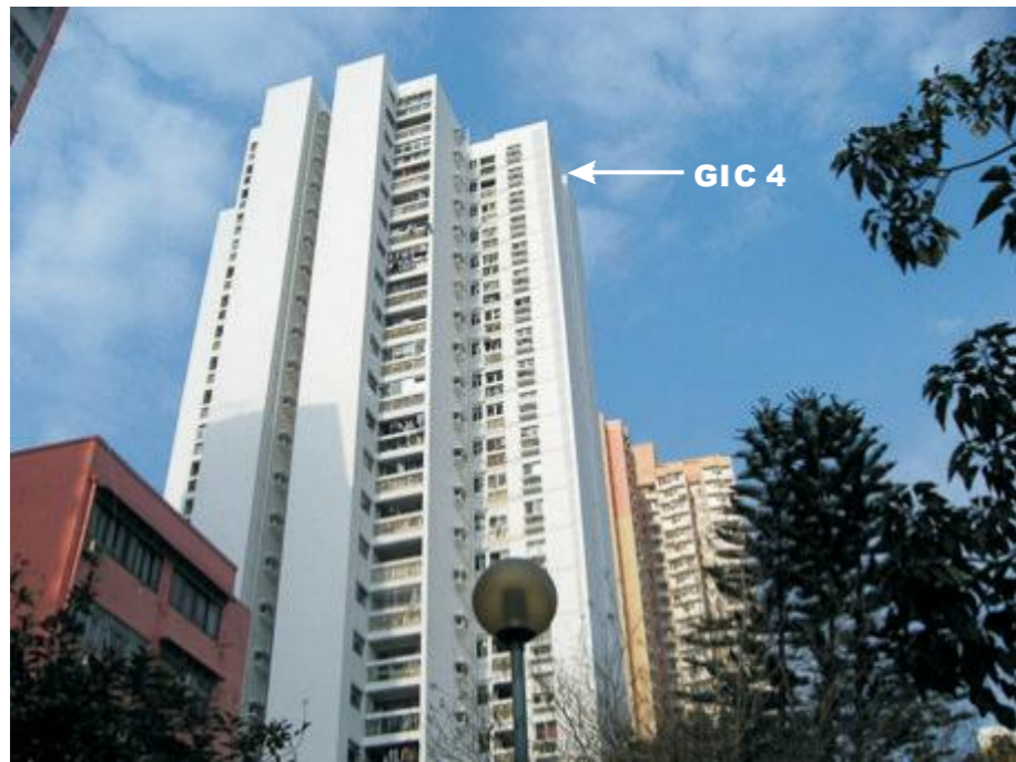
GIC4 Fire Service Department Quarters
